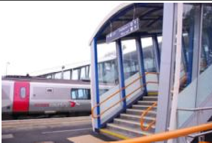
A new accessible footbridge with lifts was completed at Southampton Airport Parkway station in 2009 as shown here (new footbridges were also installed at Fareham and Fratton)
